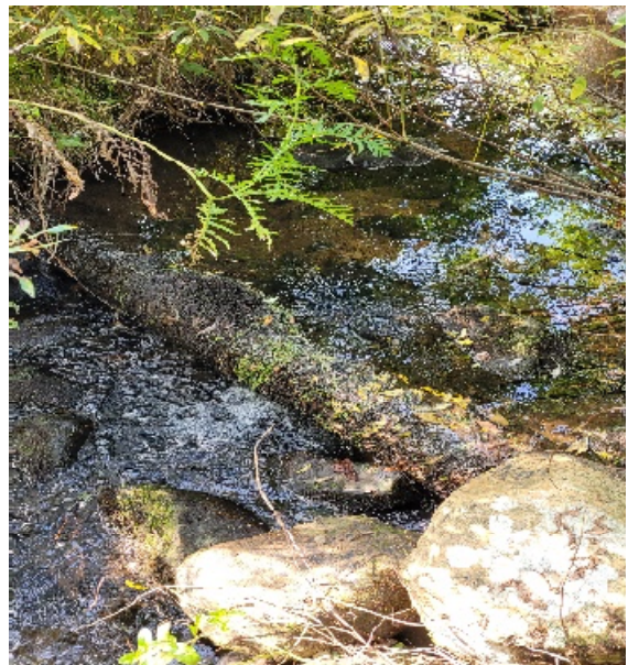
Photo 1: Exposed Rocky Branch Transmission Main Crossing
